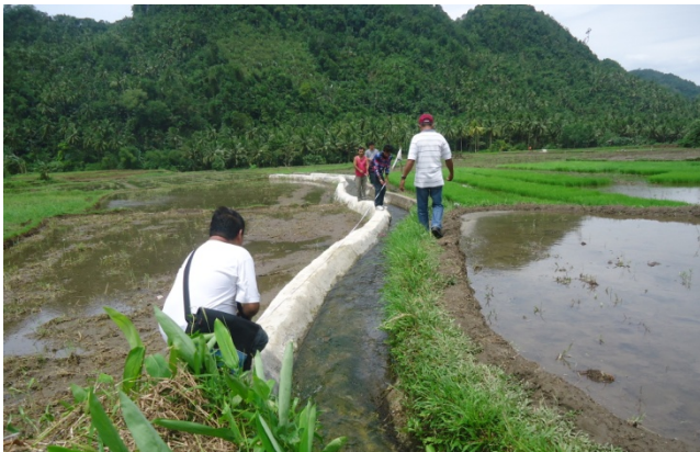
POWERS volunteers inspecting an irrigation project
